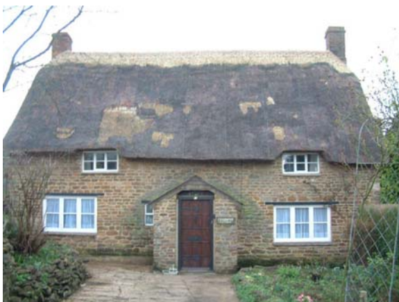
A full re-thatch is not always required with localised repairs sustaining the life of the roof.
