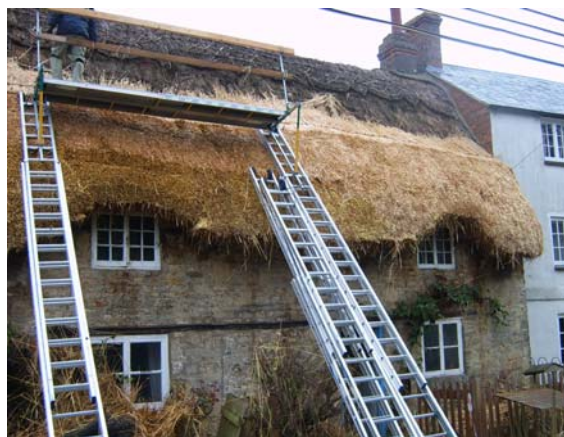
Spar-coating onto an existing thatch coat starting from eaves and moving up to ridge.
