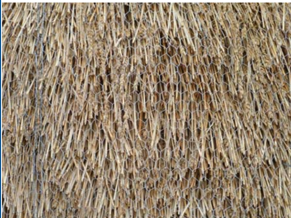
Netting is a characteristic of long straw roofs but needs to be applied carefully.
