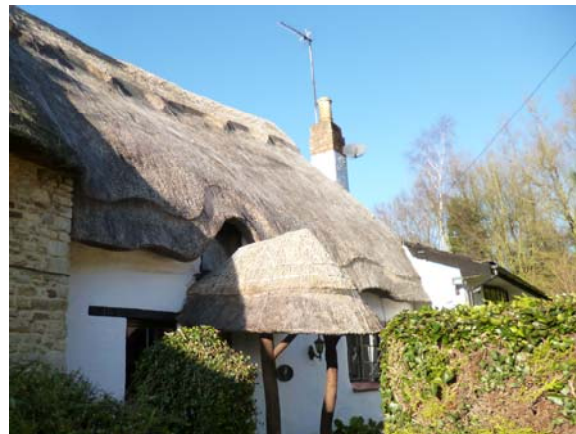
Example of a water reed thatched roof with a combed wheat block cut ridge
