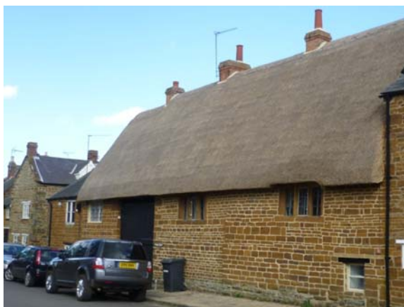
Example of a newly thatched combed wheat roof with flush ridge
