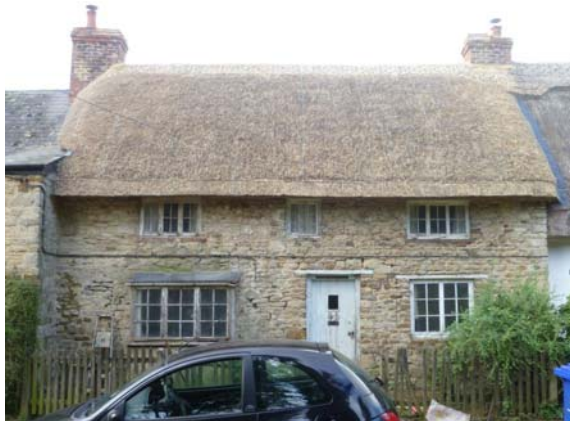
Example of a recently thatched long straw roof with a traditional flush ridge with decorative cross spars.
