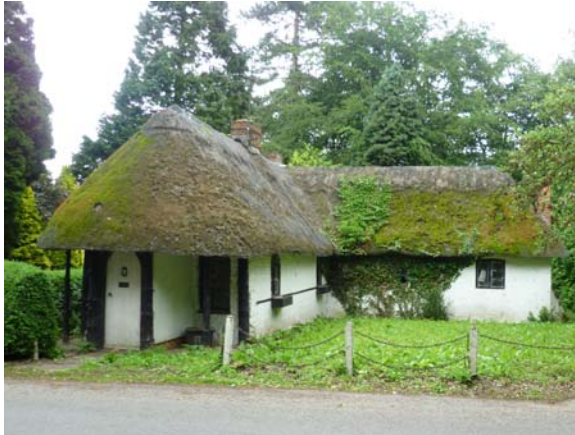
Overhanging trees, creeping plants and vegetation can all cause damage to thatched roofs.
