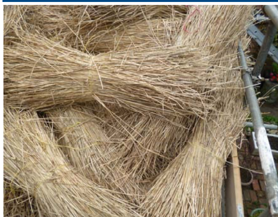
Yealms of long straw, clearly showing the intermixture of butts and ends
